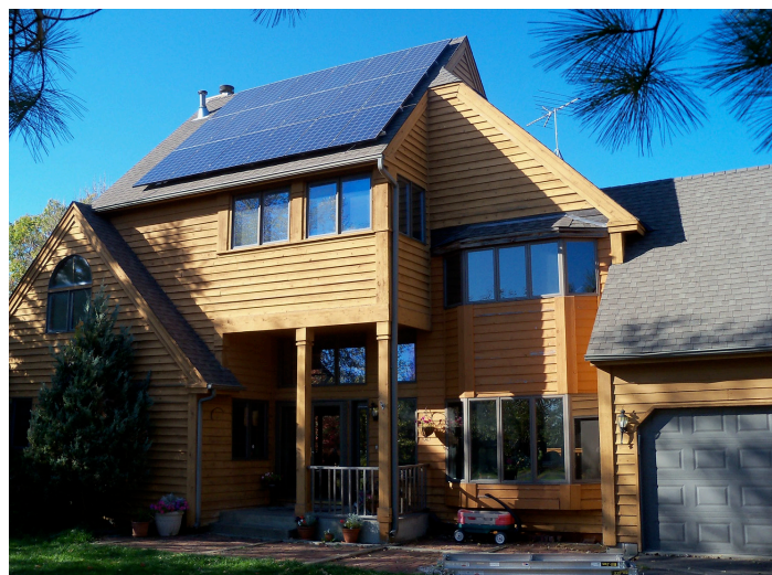
Residential PV solar installation in Minnesota
